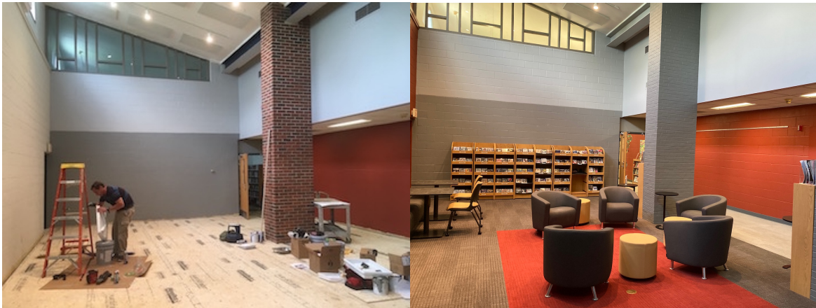
Community Room Before and After:
